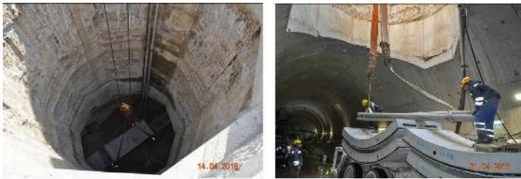
Figure 10. Loading materials on an MSV through the logistic shaft.
