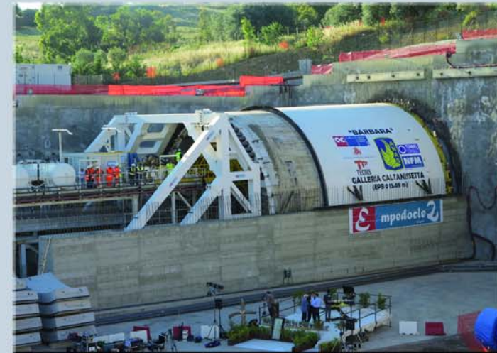
Caltanissetta highway tunnels Sicily
