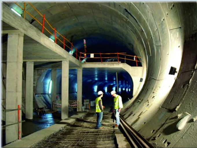
Barcelona Metro - Line 9
