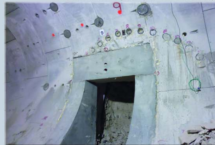
Aked Tunnel N1
